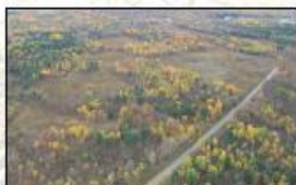
Aerial view of the clear-cut blocks in Training Area 14E looking south down U.S. Military Highway on Fort Drum. In this area, approximately 140 acres was divided into 5 acre blocks with a plan to harvest one-third in a patchwork or mosaic of blocks every 15-20 years. The first third was harvested in 2005-2006 and the second third was harvested in 2019-2020.
